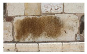
Figure 15. Abrasion on stone surface due to chemical effects
