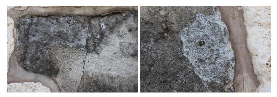
Figure 14. Defects caused by air pollution and exhaust gases
