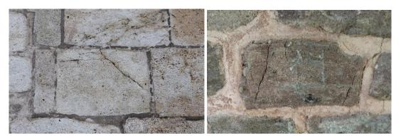
Figure 12. Crack - fracture formations on the stone surface
