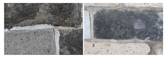
Figure 13. Crack formation in joints due to thermal expansion
