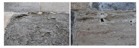
Figure 17. Abrasion on stone surface
