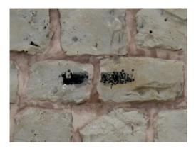
Figure 18. Pollution caused by paint and similar marking tools
