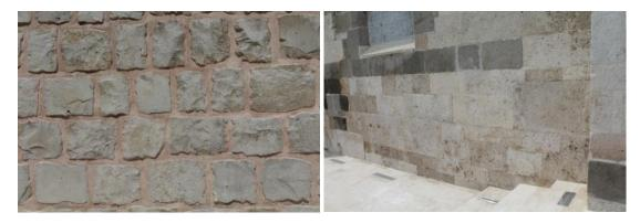
Figure 3. Facade cleaning carried out on the mosque's east facade and north courtyard facade rough masonry stones
