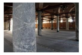
Figure 7. Surface cleaned marble columns
