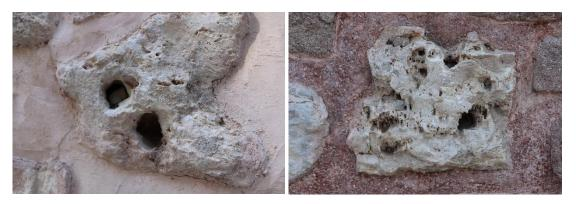
Figure 10. Macropores that occur in the formation of the stone appear as holes on the surface
